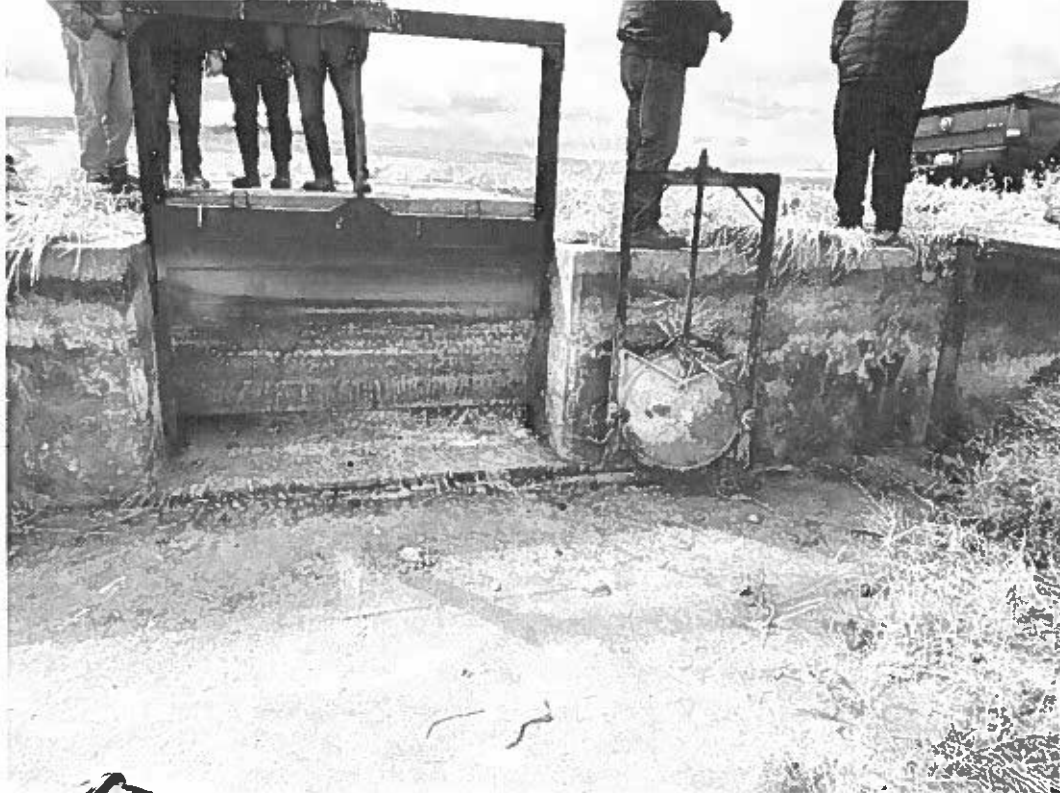
Picture 3: Existing Humbug Diversion structure
