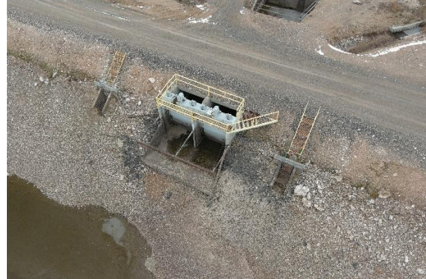
Figure 3 Aerial view of W39.9 headgate
