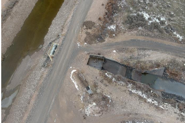
Figure 2 Overhead view of W39.9 headgate and start of lateral
