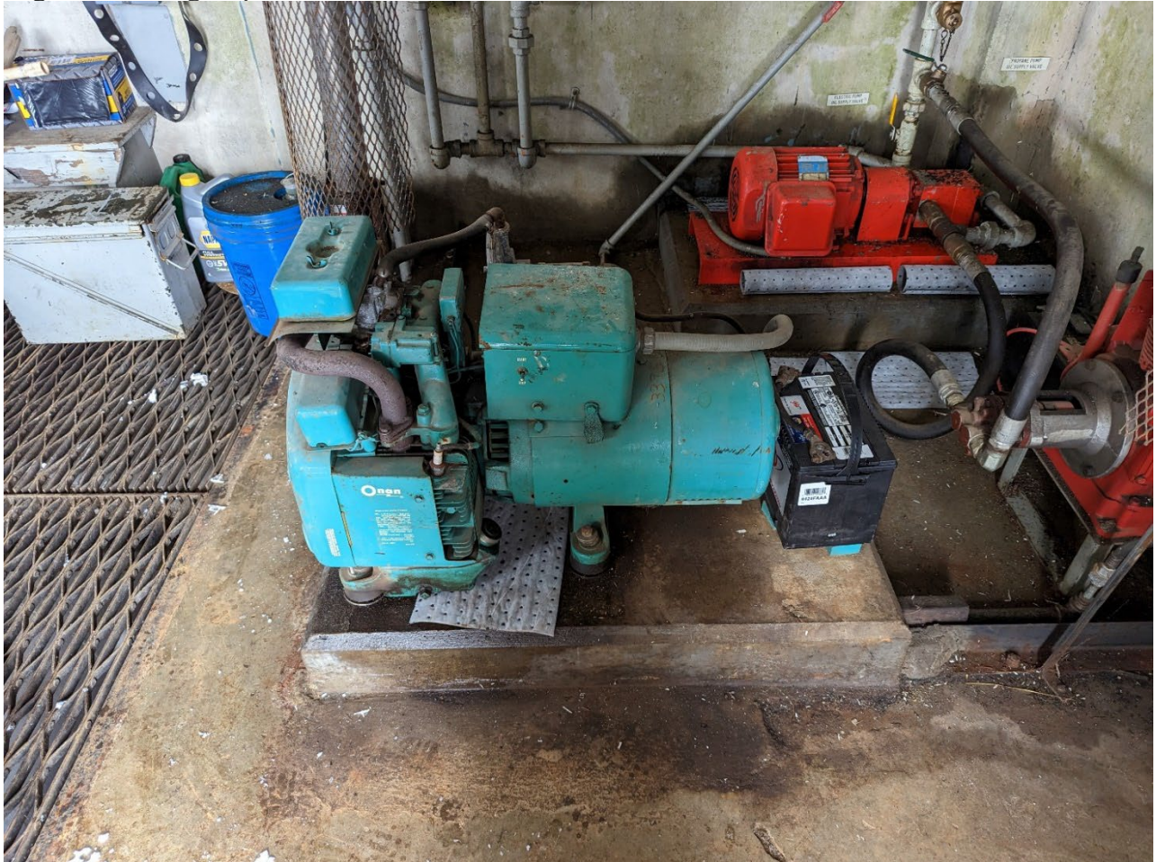
Figure 1-Existing Propane Generators
