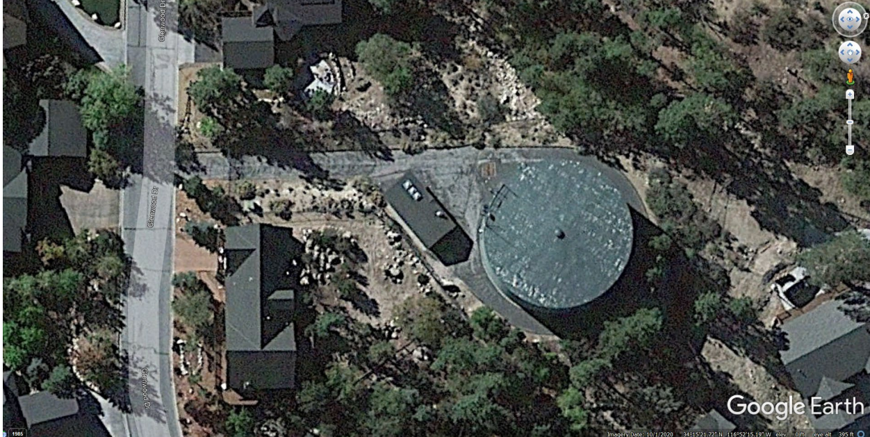
Figure 2 Existing Pontell Booster Station
