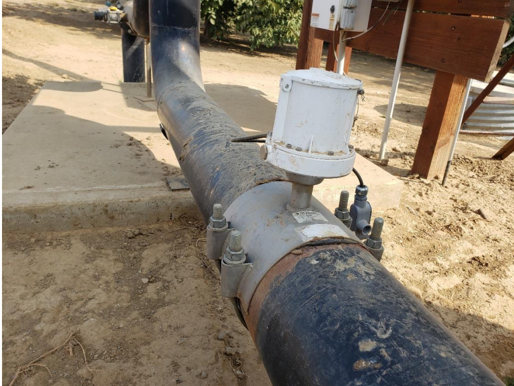
Figure 4: Typical Flowmeter Installation
