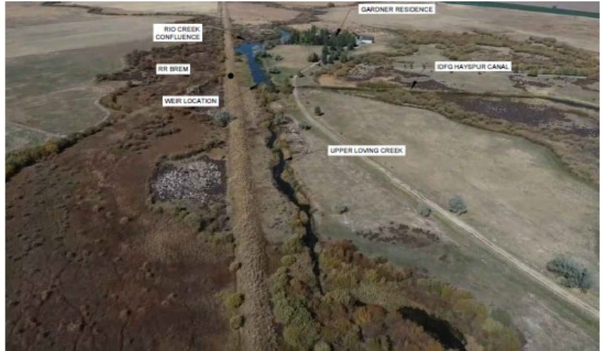
Figure 3: 2022 Aerial of Phase 1 Project Area, Looking North
