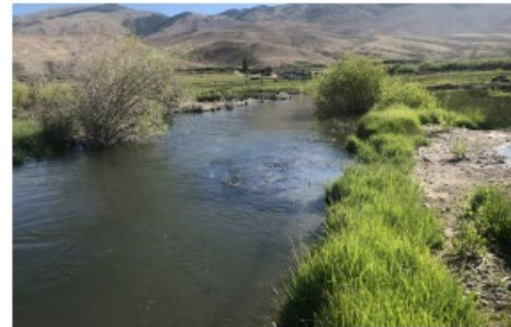
BELOW: BANK FILL WITH WETLAND SOD BANK 1-YEAR POST-CONSTRUCTION (LENNY RIVER, ID)
