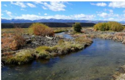
ABOVE: BANK FILL WITH WETLAND SOD BANK IMMEDIATELY AFTER CONSTRUCTION (BIG SPRINGS CREEK, ID)
