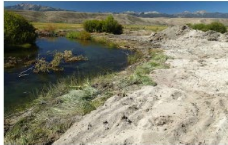
ABOVE: WETLAND SOD BANK IMMEDIATELY POST-CONSTRUCTION (BIG SPRINGS CREEK, ID).
