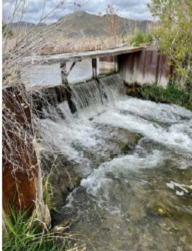
Figure 2: Irrigation Dam to be Removed
