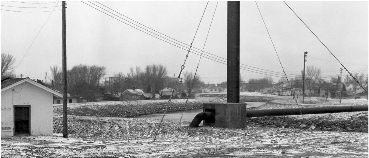
Figure 5: View of the Levee looking Northeast.
