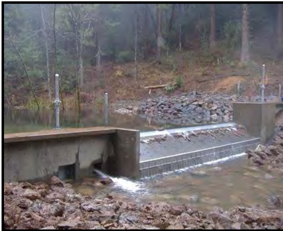
Figure 2: Coanda Fish Screen example.
