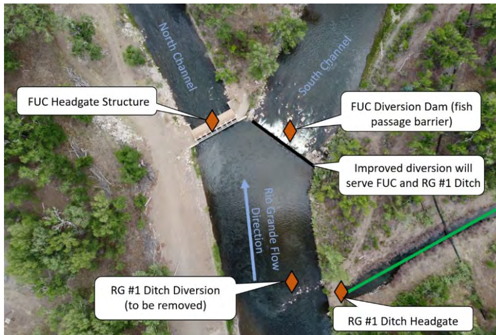
Figure 3. Aerial photo of diversion infrastructure bifurcating the Rio Grande.
