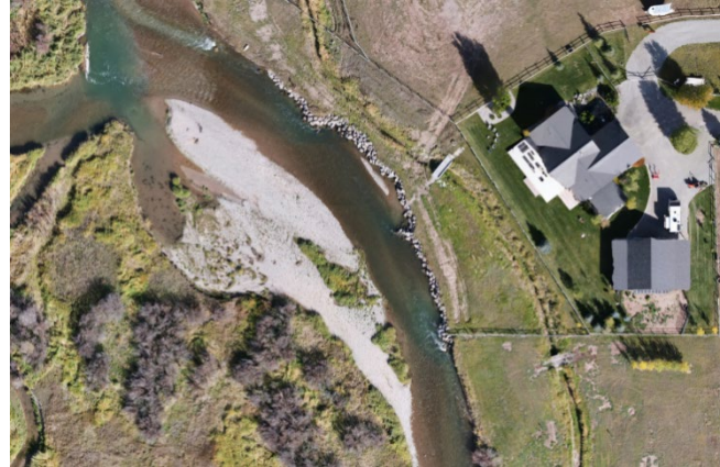
Photo 4: Channel instability in the Rico Diversion project reach. The channel migrated by at least a full channel width during 2023 runoff before NRCS Emergency Watershed Protection funds were used to place riprap to protect infrastructure. Freshly aggraded sediment is indicative of high bank erosion and channel migration.
