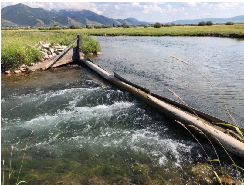
Figure 5: A log and plywood dam used for irrigation impairs stream function and proper routing of sediment and is a likely barrier to upstream fish passage.
