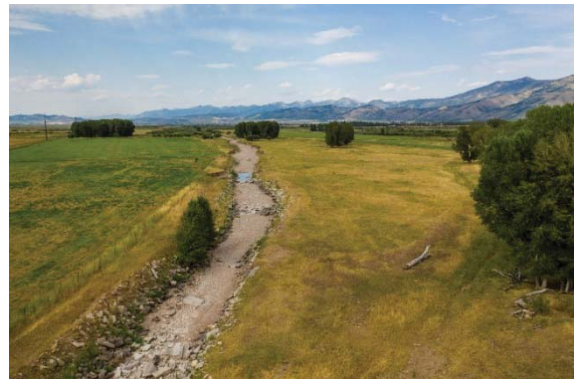
Figure 9: A channelized, riprapped reach of the seasonally dry section of the mainstem Salt River does not allow for floodplain access and results in sediment deposition downstream in the blue ribbon section of the fishery.
