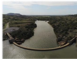
Altus Dam, Lugert-Altus Reservoir.
