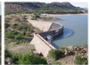
Mountain Park Dam, Tom Steed Reservoir.
