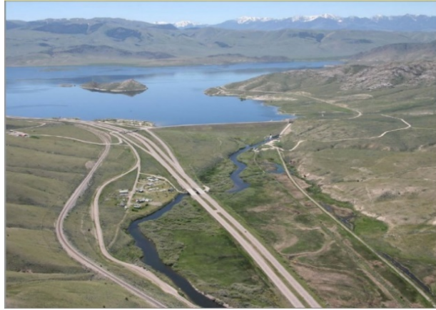
Clark Canyon Dam and Reservoir.
