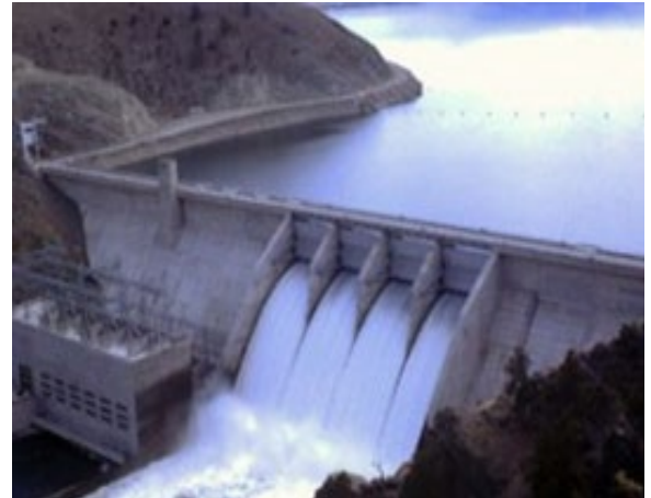
Canyon Ferry Dam.
