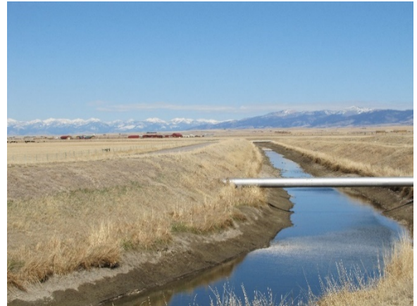
East Bench Irrigation District Canal.
