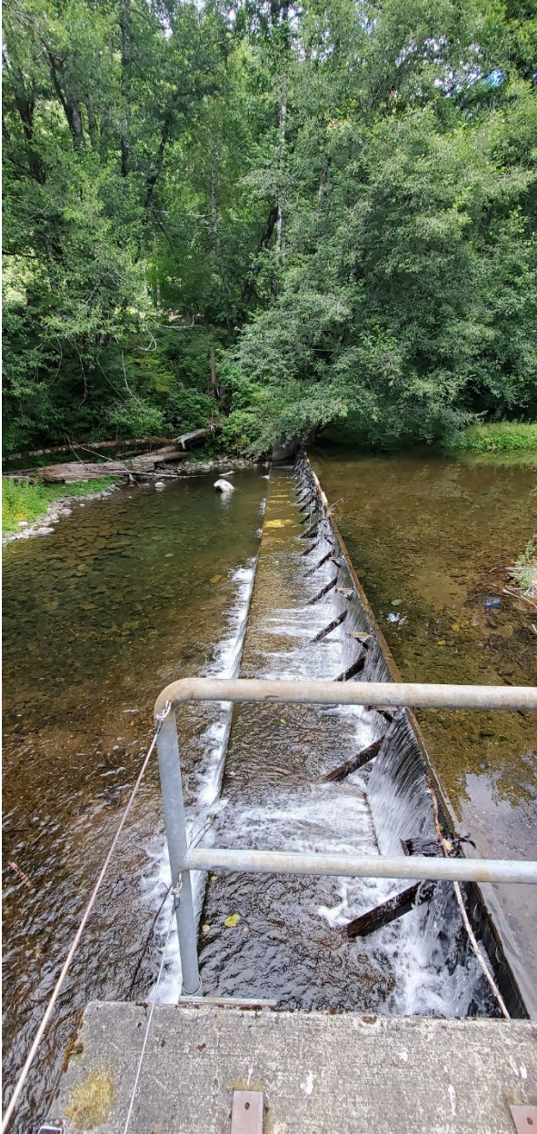
Figure 1. Tuffy Dam cross sectional view of project during low flow.
