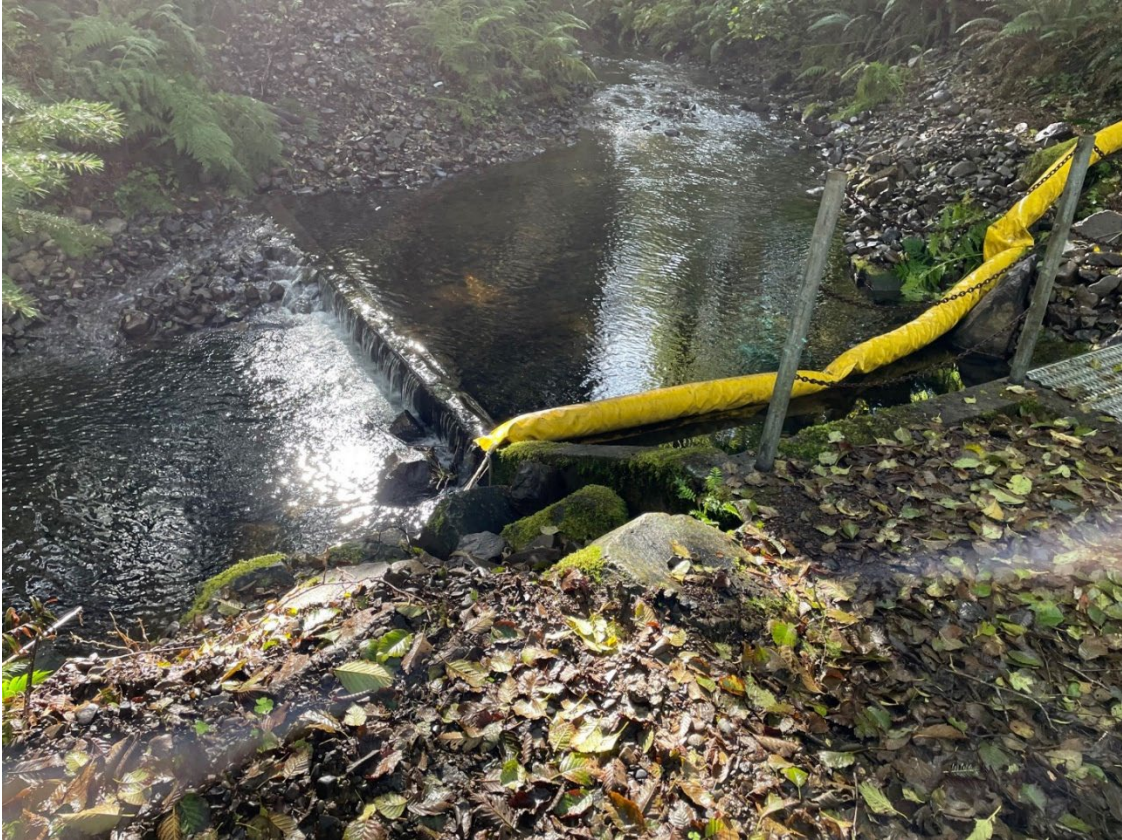
Figure 3. Cross sectional view of Whiskey Creek Dam to be removed.
