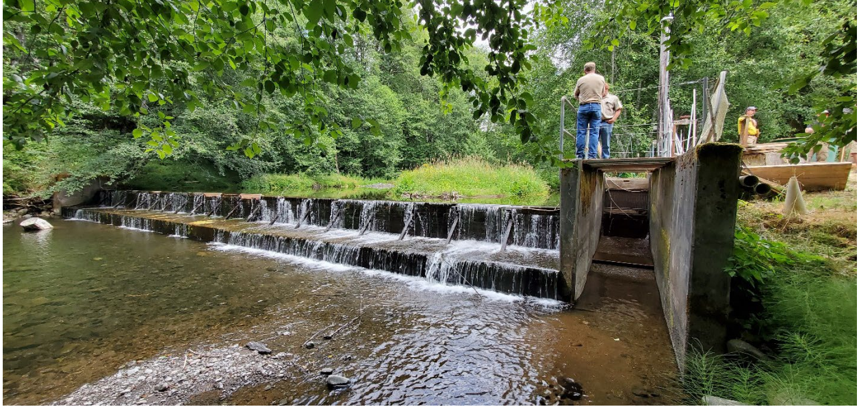
Figure 2. Tuffy Dam upstream view of dam, fishladder, and water diversion screen.
