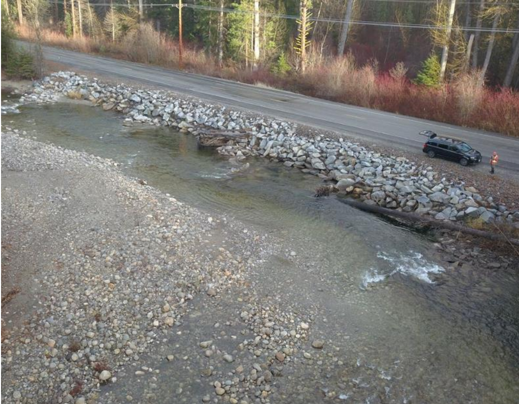
Figure 4, Rock fortified streambank with rock barbs in channel, summer 2022.
