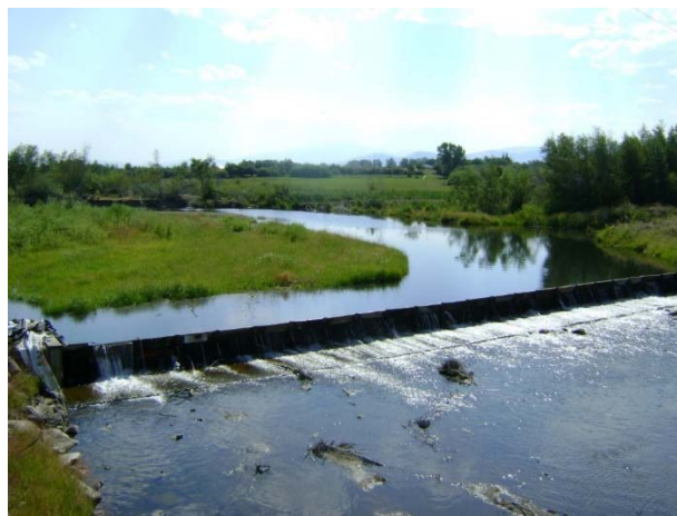
Figure 5. Sager Lane Pumps diversion dam and intake, Clark Fork River (TU photo)
