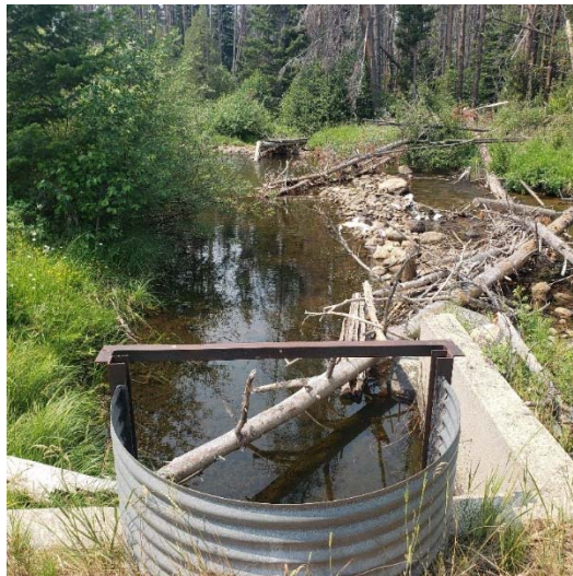
Figure 190. Ross Fork Rock Creek 1 diversion, Ross Fork Rock Creek (TU photo)
