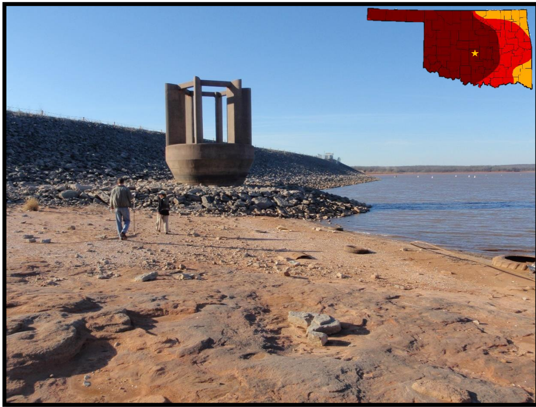
Lake Thunderbird Spillway Intake, 2013
