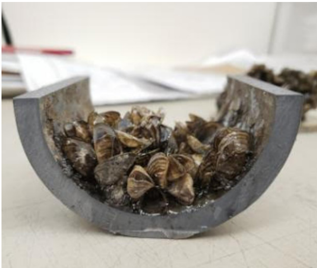
Figure 1. Example: cross-section of a pipe showing a buildup of zebra mussels
