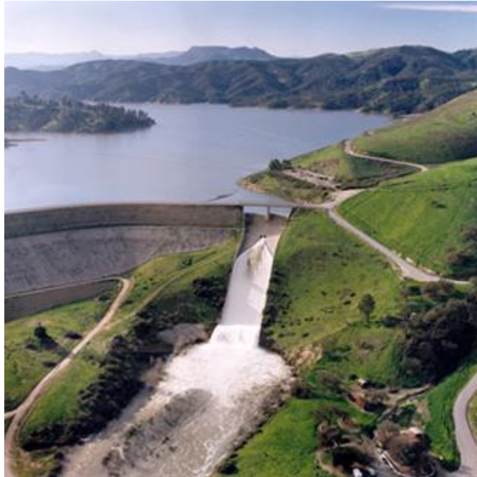
Exhibit 1. Nacimiento Dam and Reservoir
