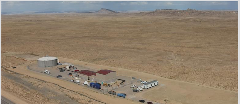
Aerial photo of Pumping Plant 3.
