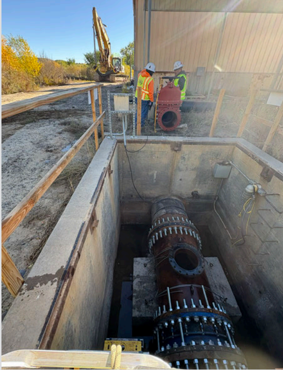
WCA crews preparing pipe for inspection.
