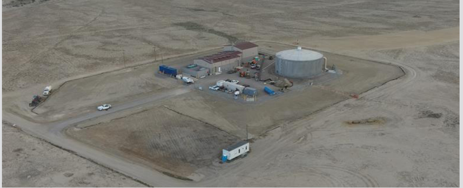
Aerial photo of Pumping Plant 2.
