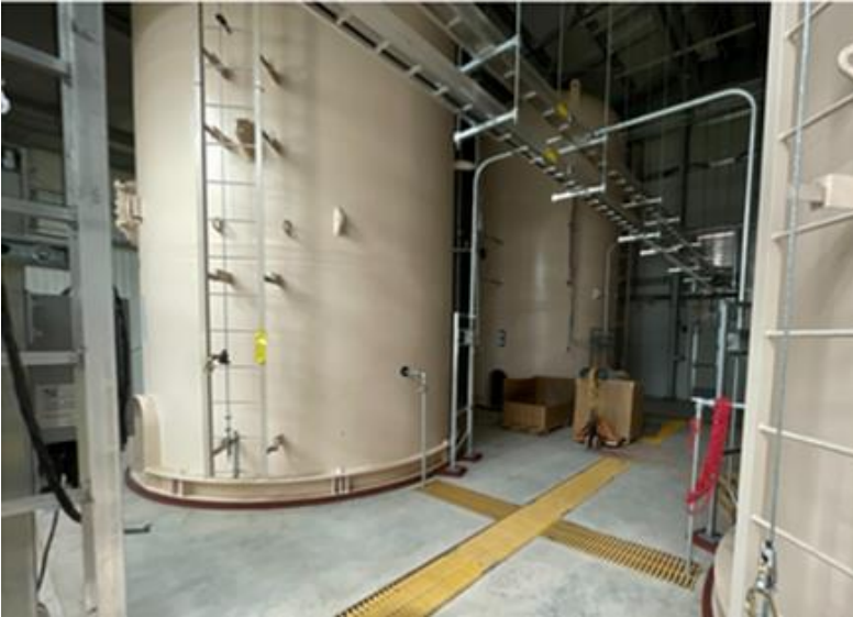
The air chamber room at San Juan Lateral Pumping Plant 4. Photo by Ed Tsosie
