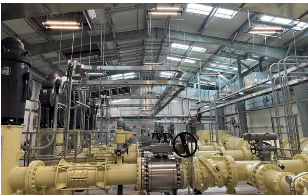
San Juan Lateral Pumping Plant 4—Pump Room Interior. (Vertical turbine pumps on the left and discharge manifold on the right.) Photo by project contractor Archer Western
