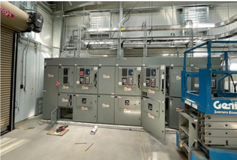
The motor control center at San Juan Lateral Pumping Plant 4. Photo by Eugene Tanner
