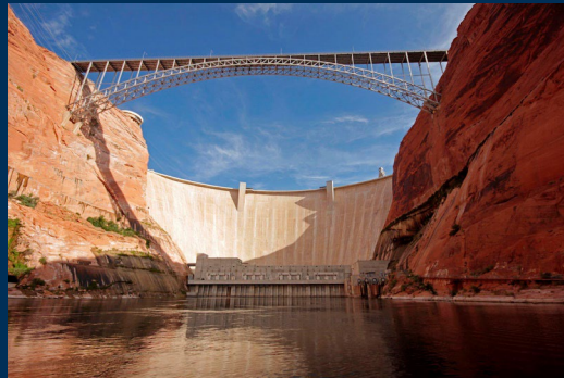
Photo: Bureau of Reclamation
