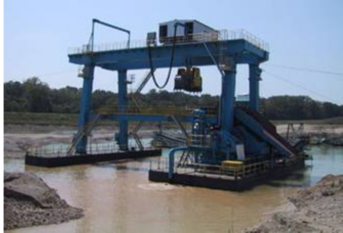
Figure 10. Clamshell dredge excavating sediment.
