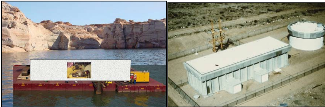
Figure 17. Pumping plants on Lake Powell would be floated on modular barges while pumping plants on land would be contained within permanent buildings.
