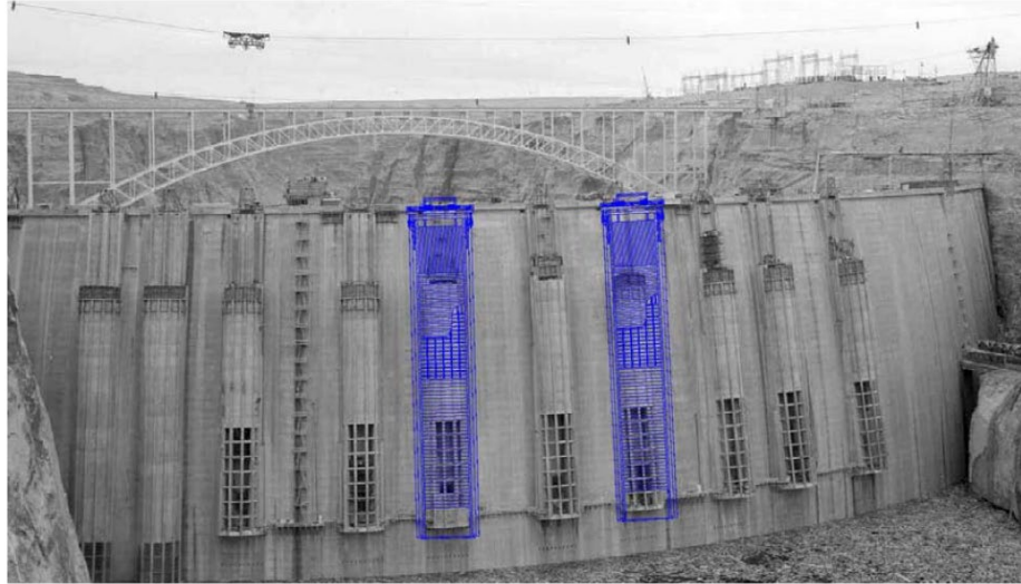
Figure 1. A construction photograph of the penstock intake structures on the face of Glen Canyon Dam. A schematic of the proposed TCD structures has been added to illustrate their proposed size and location.
