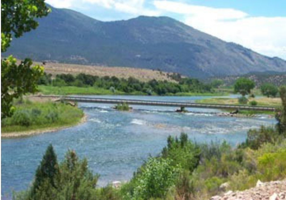
Looking North at Brown's Park Bridge.
