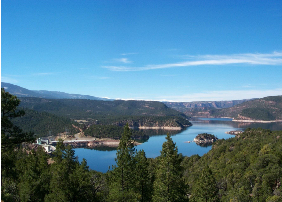
View of Flaming Gorge Reservoir from above Dam.
