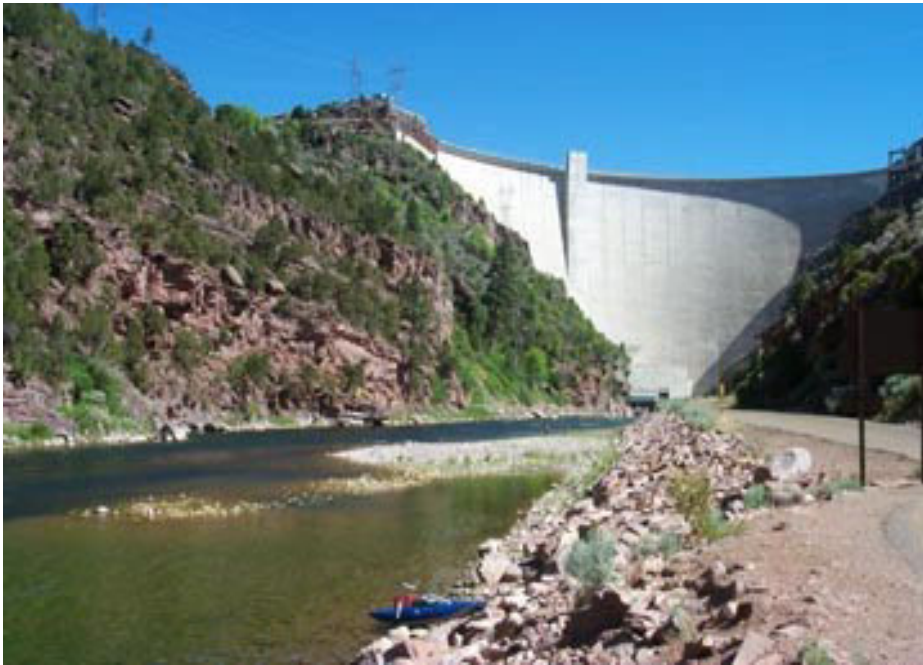
View of Flaming Gorge Dam from Spillway Launch Ramp.
