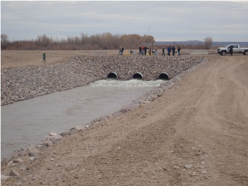
Figure 20: RM 60 looking upstream along the outfall channel toward the gated culvert structure (Reclamation, 2023)
