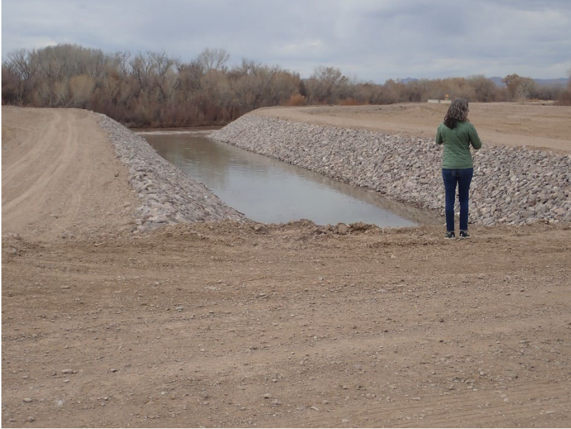
Figure 19: RM 60 looking down the completed open outfall to the river (Reclamation, 2023).
