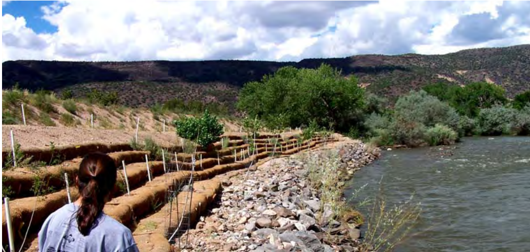
Figure 3. Bioengineered bankline at La Canova
