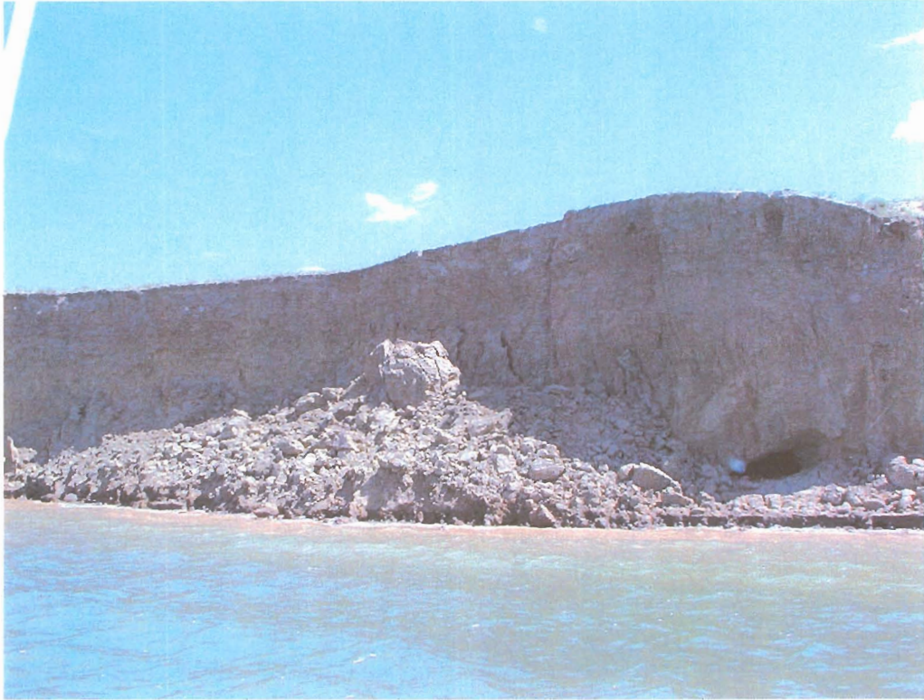
Figure 8 – Recent Eroded Material That Has Not Moved Further Into Reservoir.
