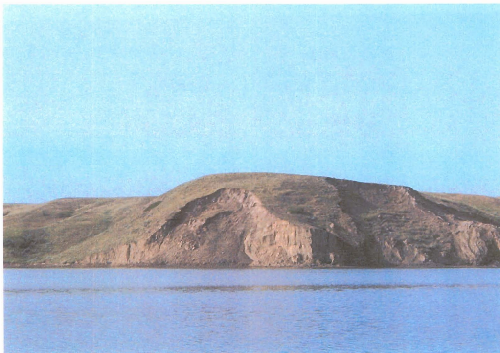
Figure 7 – Large Areas of Erosion Occurring Above the Reservoir Maximum Water Surface.
