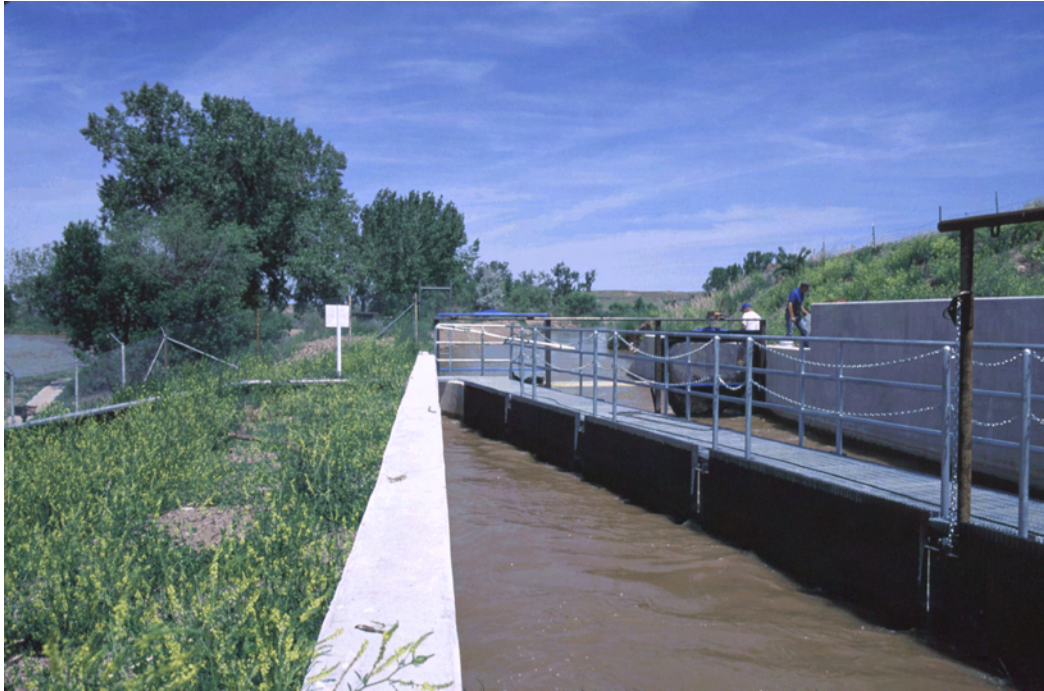
Figure 123.—Louver and walkway. Note river on the left and canal downstream beyond the louver – Example 4 (T&Y Irrigation District).
