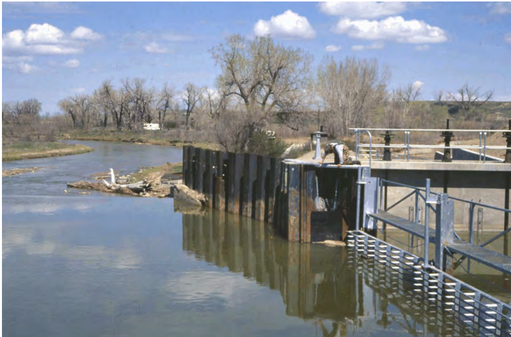
Figure 118.—T&Y Diversion Dam trashrack structure – Example 4 (T&Y Irrigation District).
