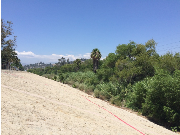
Figure 10. View of the LA River approximately 3 miles north of downtown Los Angeles. The soft-bottomed portion of the trapezoidal channel was heavily vegetated.
