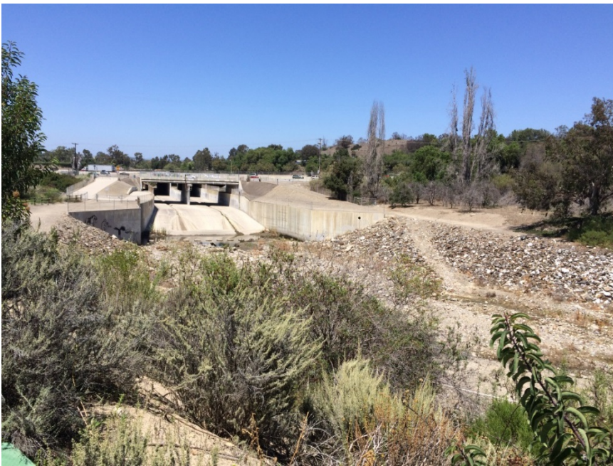
Figure 8. View of concrete drop structure looking upstream.
