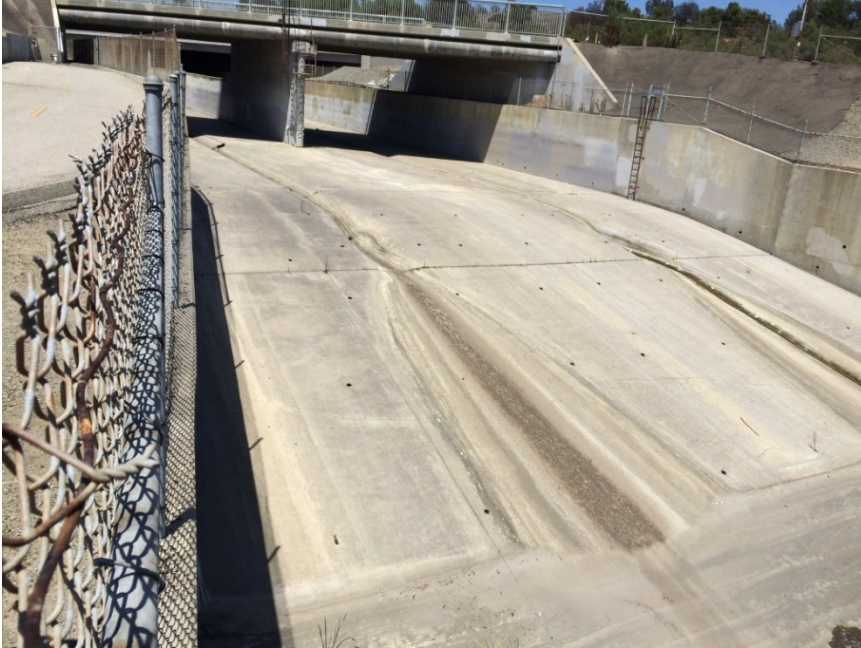
Figure 7. Upstream concrete drop structure produces an impassable fish barrier.
