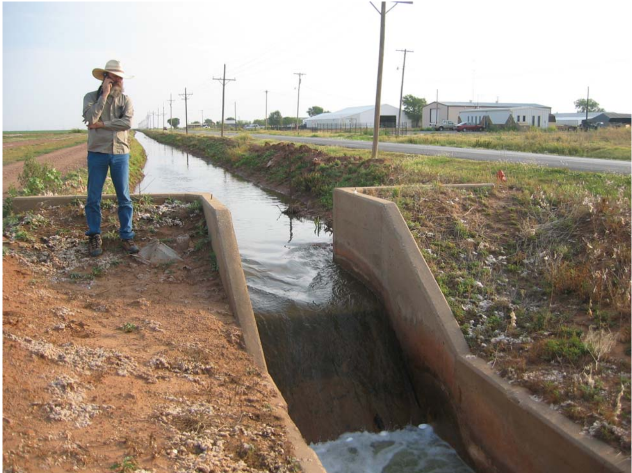
Figure 3. — Drop structure in A9.9 lateral near cotton gin.
