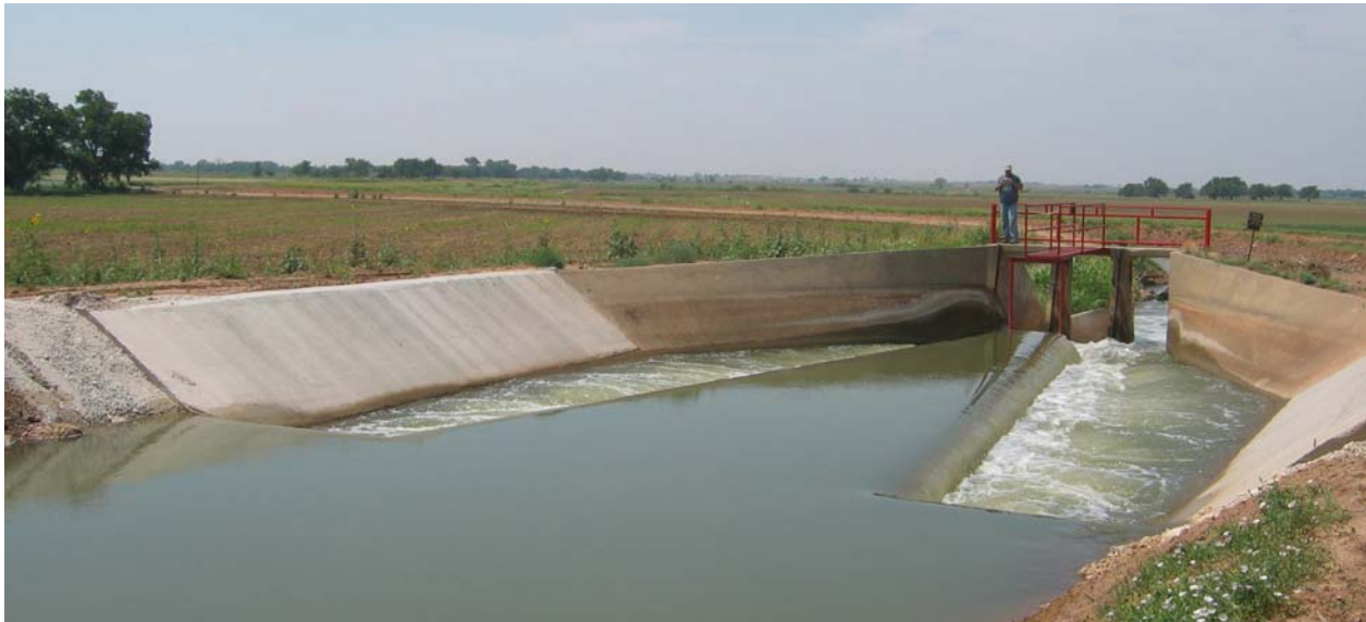
Figure 5. Long-crested weir check structure.
