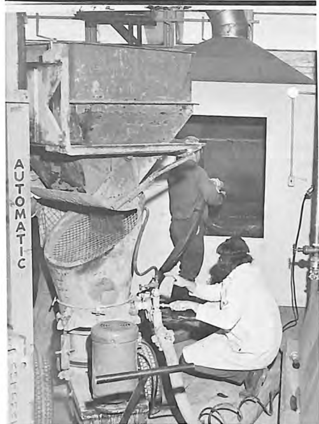
Shotcrete is applied to laboratory test panels to determine rate of set and strength characteristics.
