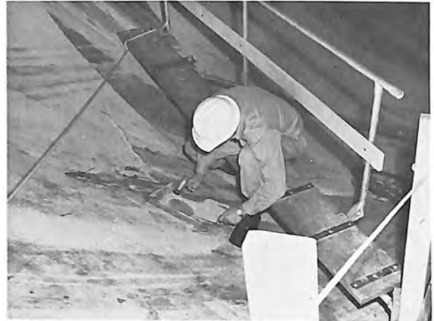
Repair epoxy mortar is being compacted using a "plastic-head" hammer.
