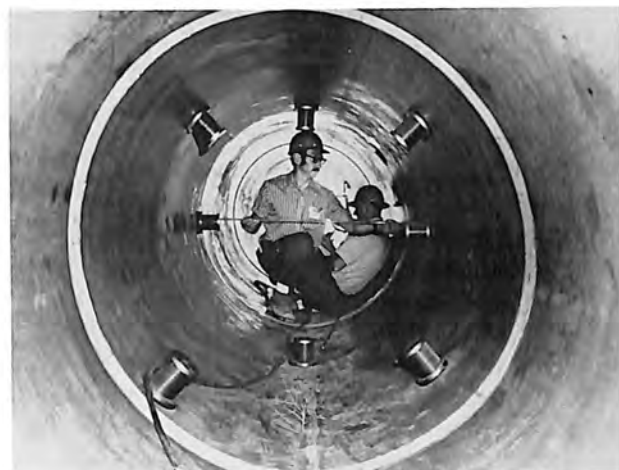
Measurement of horizontal deflections of test pipe at the E&R Center. The cylindrical projections contain cells for soil pressure measurement.
