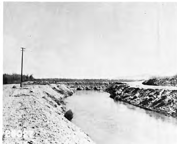
San Marcial conveyance channel, New Mexico.
