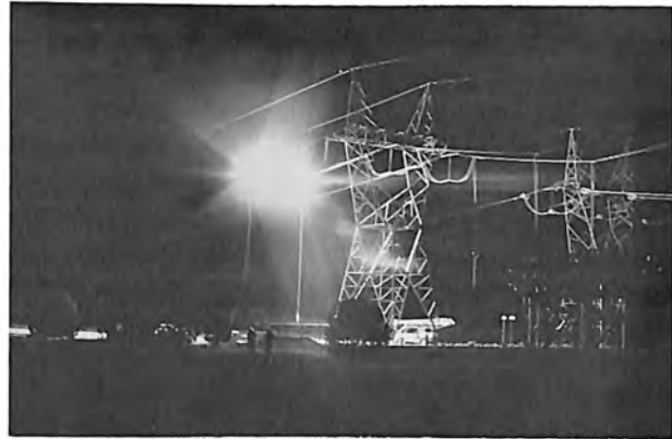
Line-to-line fault staged for Glen Canyon-Flagstaff line relay coordination checks, Colorado River Storage Project.
