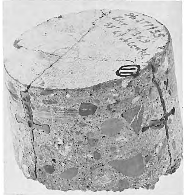
A concrete core removed from a large canal contains two PVC preformed sealing strips; the one on the left for transverse joints and the one on the right for longitudinal joints.
