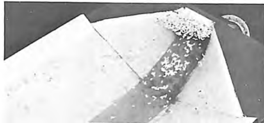
Modified inlet to the existing siphon. Photo P222-D-71735
