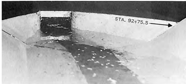
Modified inlet to the existing siphon. Photo P222-D-71744
