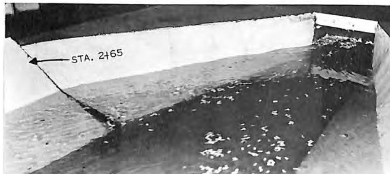
Inlet to the second siphon. Photo P222-D-71748
