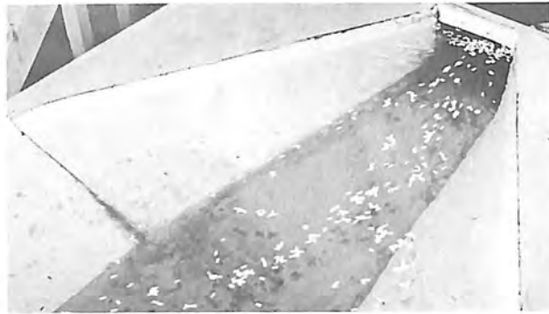
Inlet to second siphon. Photo P222-D-71734
