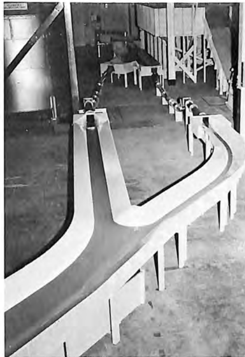
Looking upstream. Photo P222-D-71725
