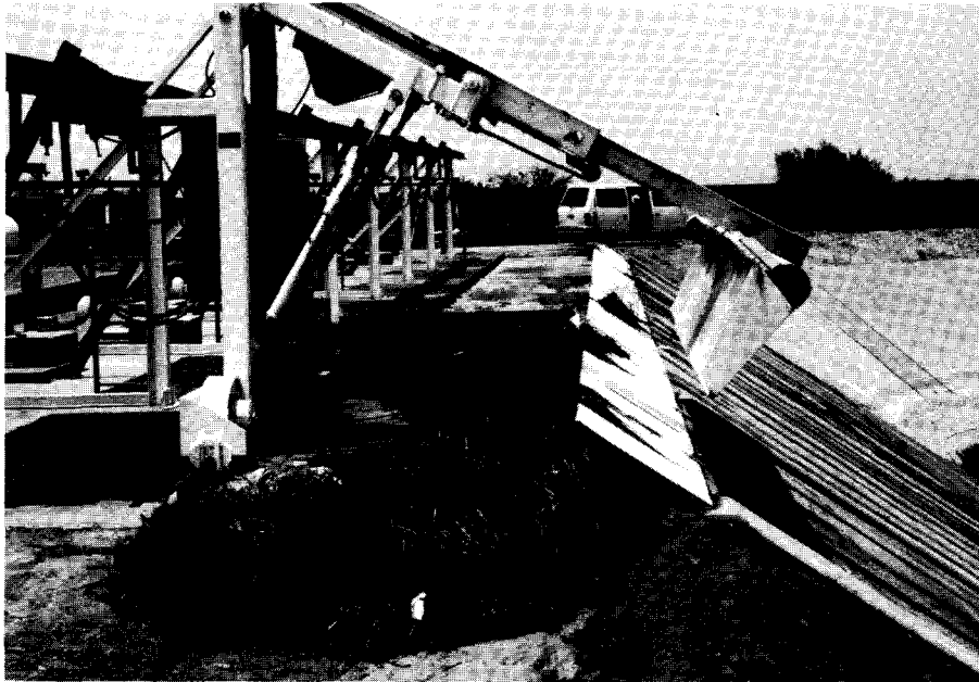
Figure 4. - Indexing hydraulic-type trash rake installed at the Santa Rosa Turnout, Arizona.
