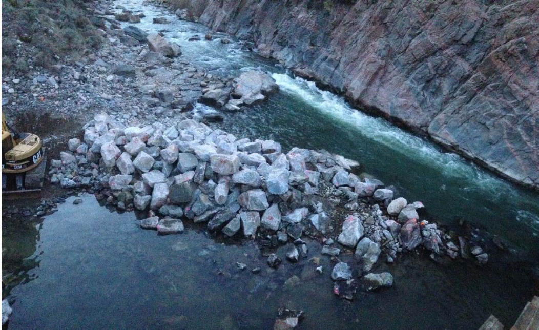
Figure 2. Photograph of tailrace protection dike repairs in 2015.
