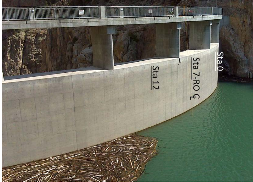
Figure 6. Photograph of Buffalo Bill Dam forebay and the stationing used during bathymetry measurements. A total of 13 sonar profiles were collected to map the reservoir bottom in the dam's forebay.
