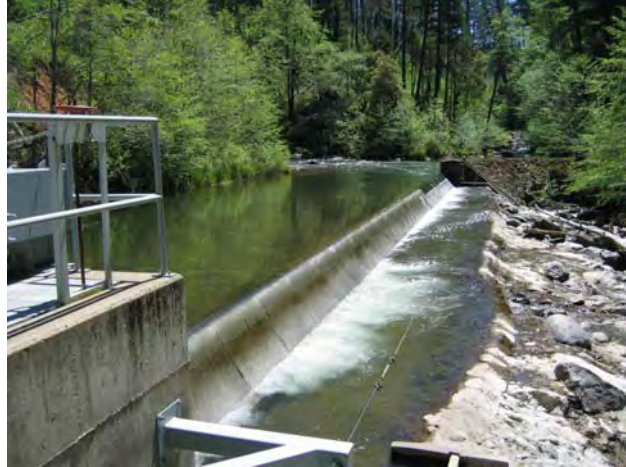
Figure 9. — Montgomery Creek intake.
