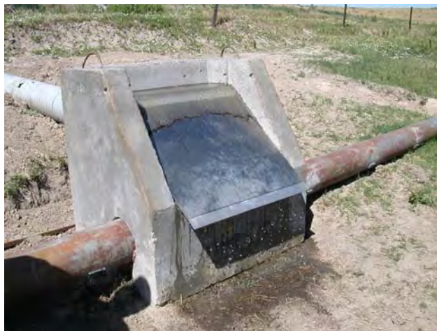
Figure 4. — Coanda-effect screen structure feeding two irrigation pipelines. Raw water enters the back of the structure through the white, PVC pipe. Screened water exits to the right and left. Overflow and debris are discharged onto the ground at the front of the screen.
