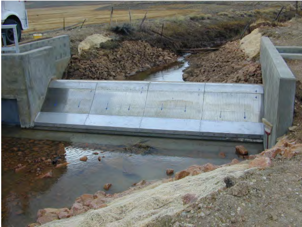
Figure 7. — Coanda-effect screen structure at Lake John, constructed in 2001. This structure replaced that shown in Fig. 6.
