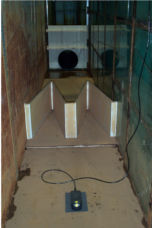
Figure 3. Looking downstream at the SW and the 0.51-m-high labyrinth weir in the open channel section. The bulkhead entrance to the 0.45-m pipe can be seen beyond the labyrinth weir. A staff gage is visible on the steel wall across from the SW transducer.
