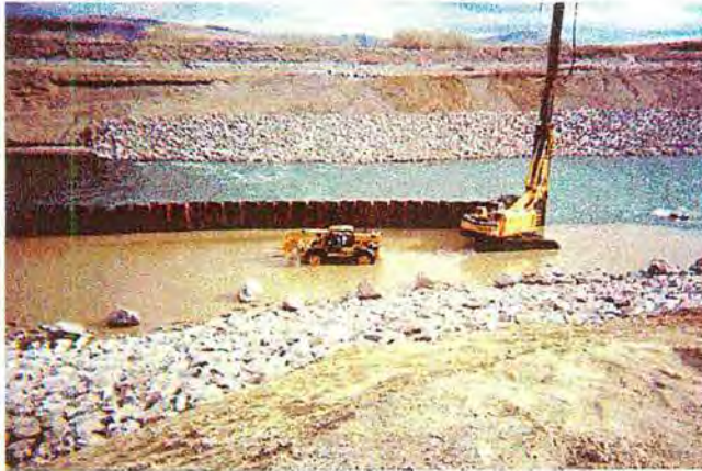
Figure 8 - Construction of Marble Bluff Dam Gradient Restoration Structure
