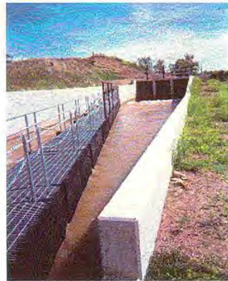
Figure 2 View of T&Y Canal Headworks and Fish Louver
