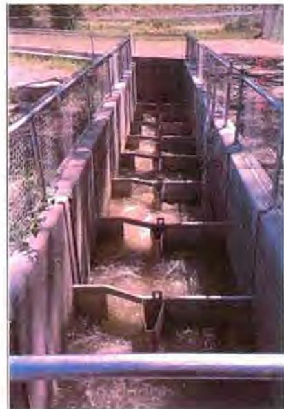
Figure 10 – View of Redlands vertical slot fishway
