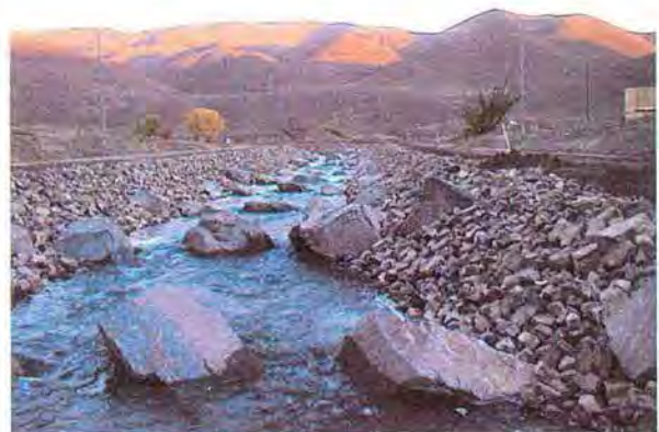
View of rock fishway looking upstream.
