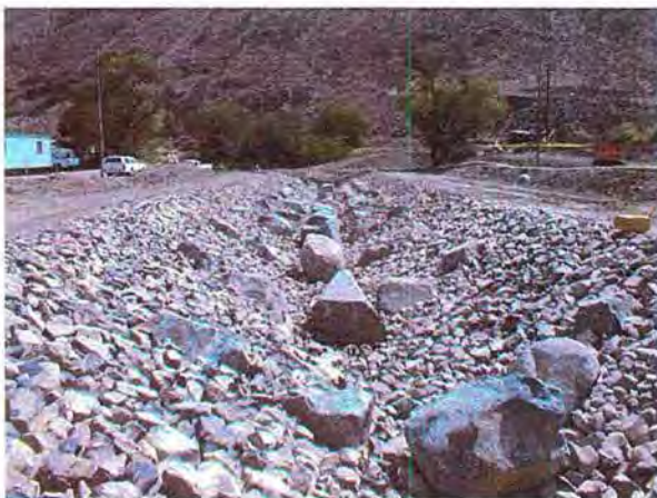
View of rock channel with boulder weirs looking downstream.
