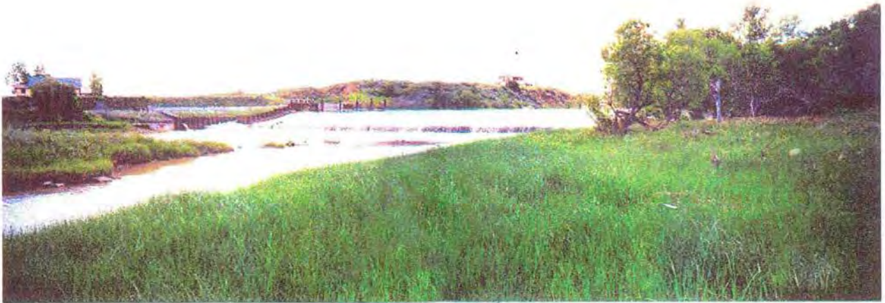
Figure 4 - View looking upstream at T&Y Diversion Dam, June 19, 2001. River flow downstream of the dam was about 200 ft 3 /s.
