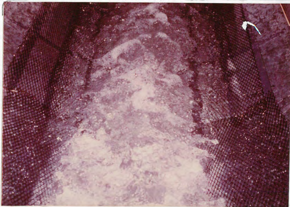
Figure 5 - Hydraulic jump at base of drop, 8.33 \text{ m}^3/\text{s} ( 294 \text{ ft}^3/\text{s} ).
