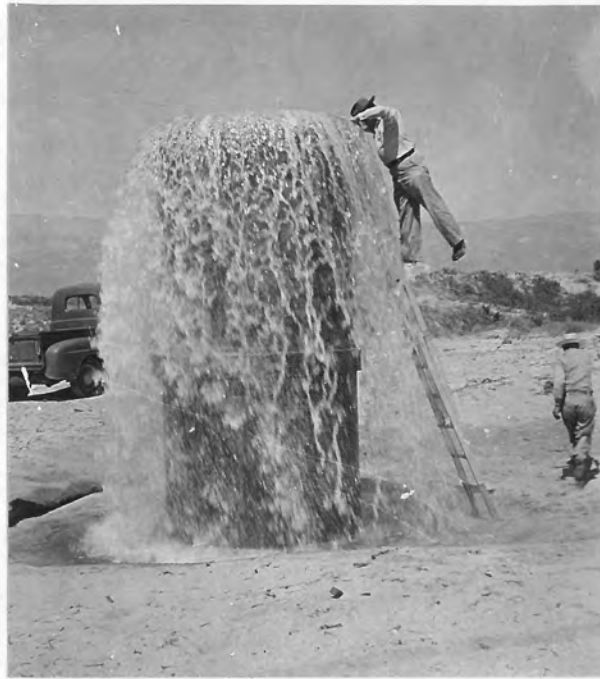
FIGURE 4. OVERFLOWING PIPE STAND--COACHELLA DISTRIBUTION SYSTEM, CALIFORNIA
