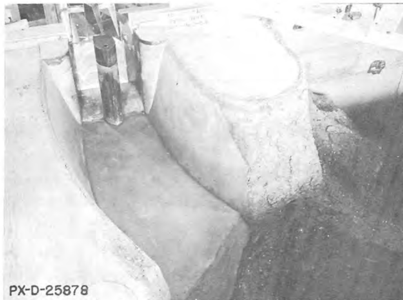
A. Reservoir area and spillway entrance structure.
