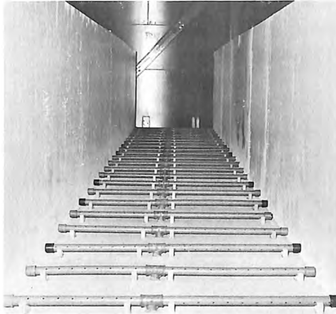
A. Drainpipes in bottom during fabrication of seepage tank. Photo PX-D-60404
