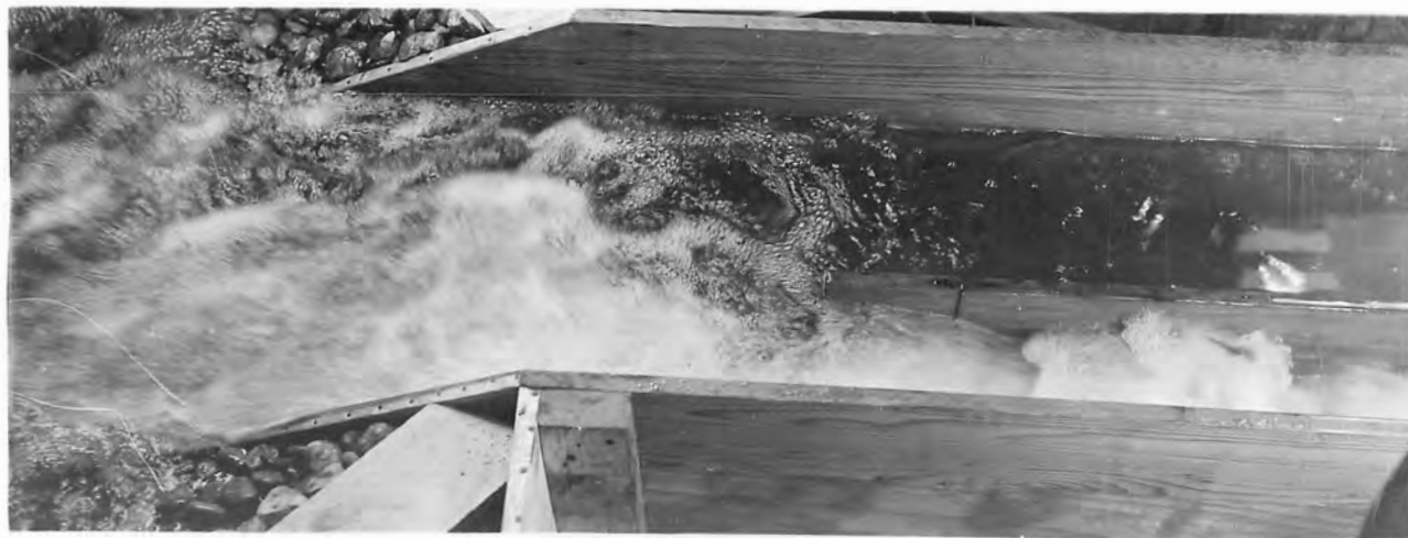
C. RECOMMENDED DESIGN; LEFT VALVE 1975 SECOND- FEET.
