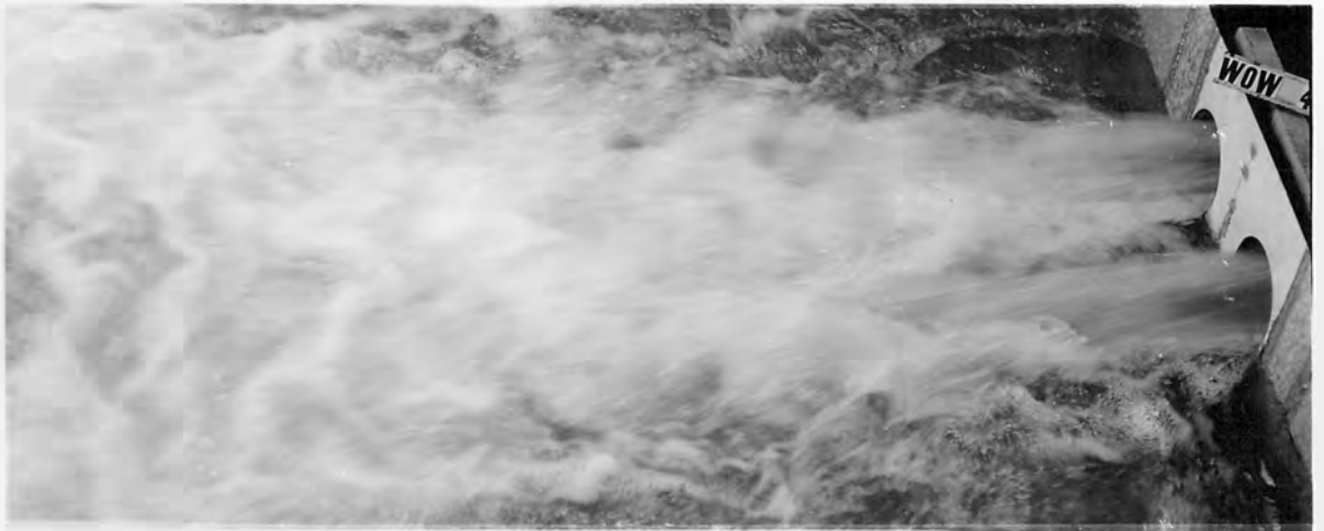
B. 3950 SECOND-FEET; VALVE CENTERLINE EL. 4263; TAILWATER EL. 4264.4.
