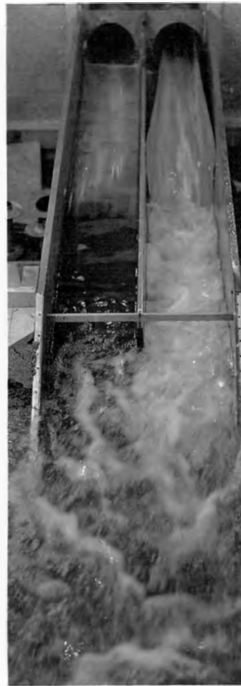
C. 1975 SECOND-FEET; FLARED CHUTE WALLS.
