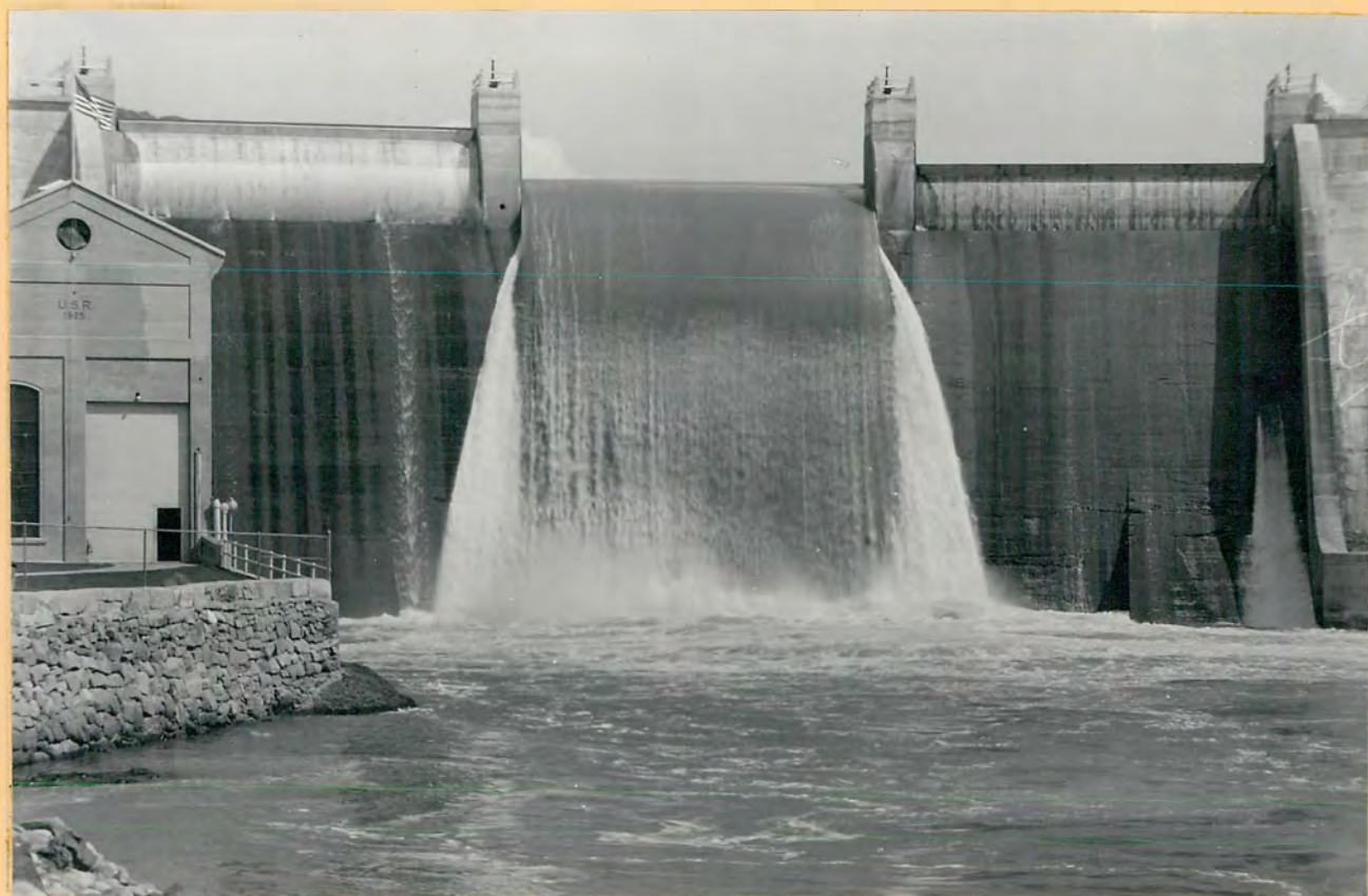
B. Gate Completely Lowered - Head on Gate 7.7 Feet Showing Spread of Jet on Face of Dam
