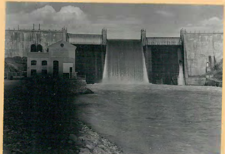
D. Gate Completely Lowered - Head on Gate 9.1 ft.
