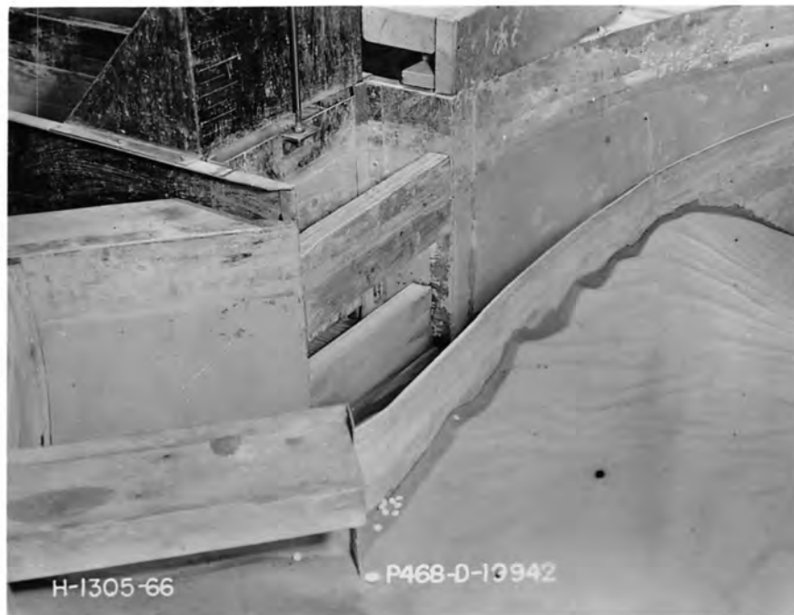
(a) Stop logs in place below curtain wall
