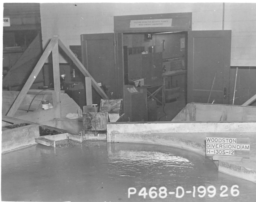
(a) Looking downstream towards headworks and sluiceway
