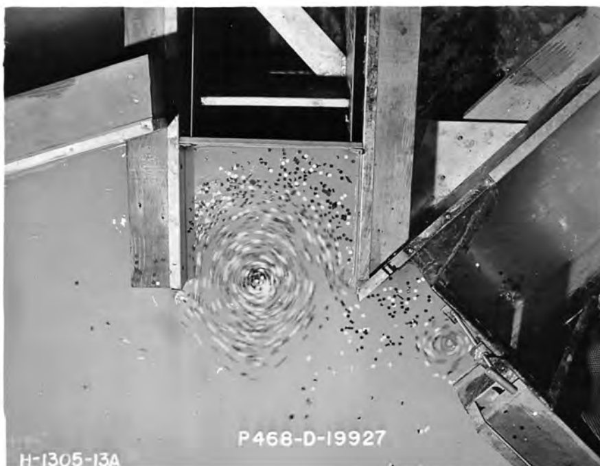
(b) Vortices in front of sluiceway and headworks
