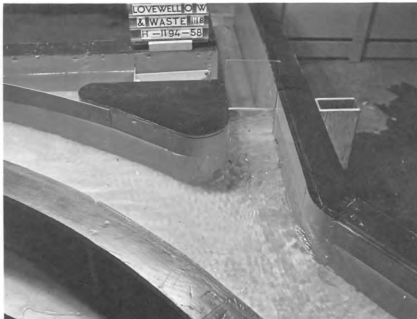
A. Original Wasteway Entrance Closed by Curved Wall and New Entrance Provided Downstream.
