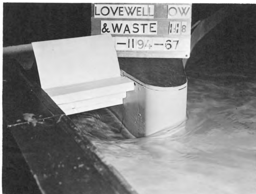
B. Gate Fully Opened. Water Surface Elevation at Canal Inlet--1570.10.
