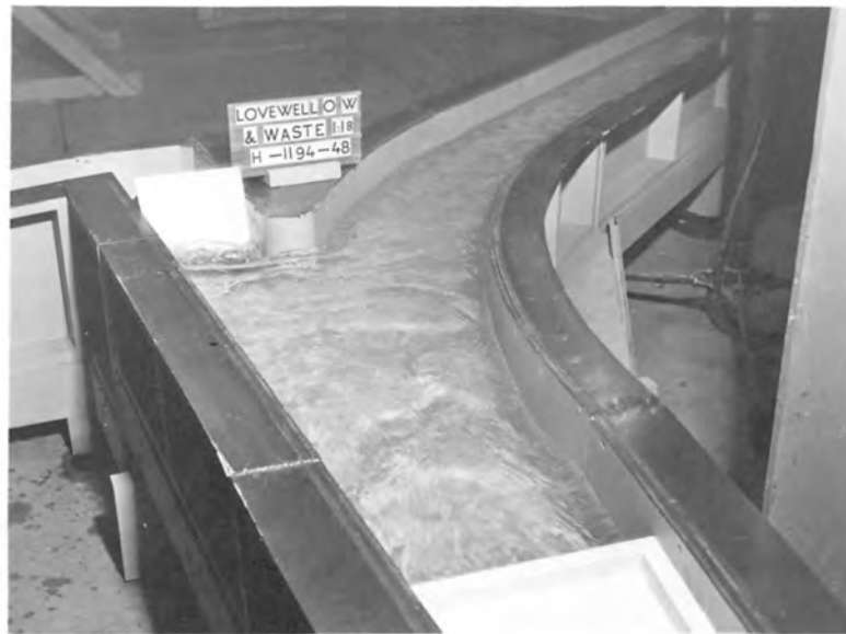
C. Y-Section 635 cfs Released by Wastegate and 635 cfs in Canal Supply Channel.
