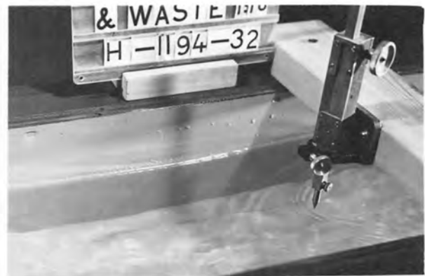
Canal Supply Channel--Station 7+55. 00 Note curve in water line on sidewall.
