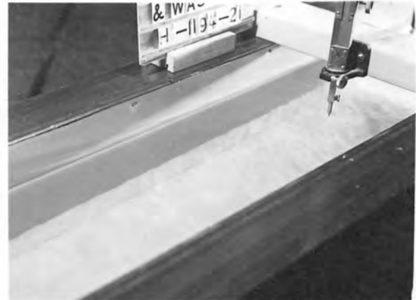
Canal Supply Channel--Station 7+55. 00
