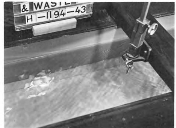
Canal Supply Channel--Station 7+55.00
