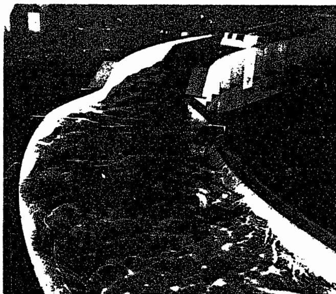
Without suppressor - waves overtop canal.
