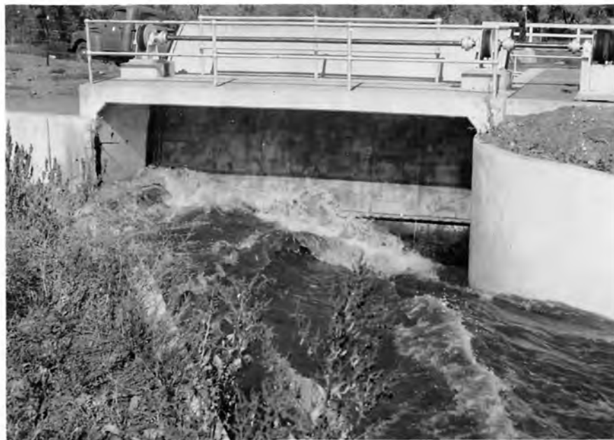
B. Water Surface Drawdown at radial gate.
