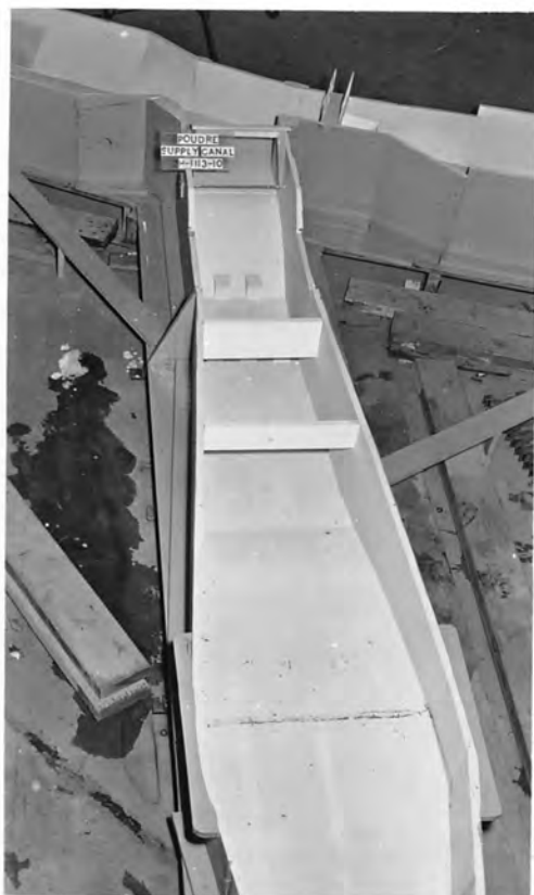
A. Curtain walls looking up-stream.
