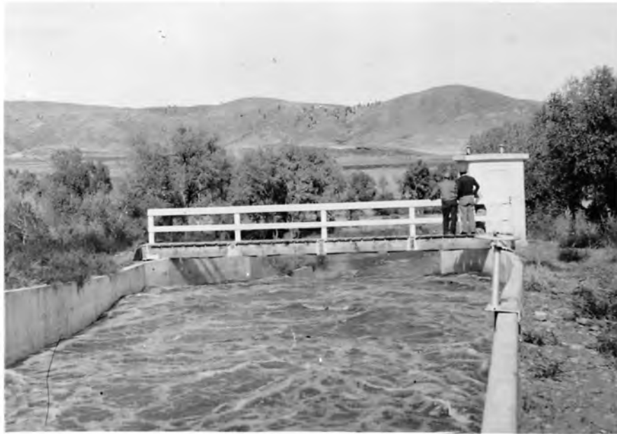
A. Looking downstream in Measuring Flume. The water surface fluctuation averages about 10 inches with a maximum of 18 inches.
