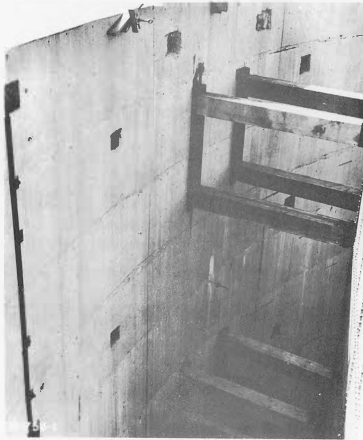
A. TIMBER WEDGE STRUTS BETWEEN TIPPING SECTION AND MITER GATE LEAVES.
