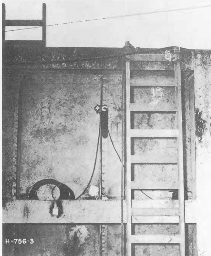
A. PRESSURE CELL INSTALLATION-MITER GATE EL. 957.81
