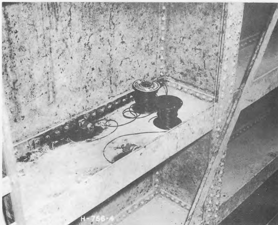
B. PRESSURE CELL INSTALLATION-MITER GATE EL. 942.33 & 922.58
